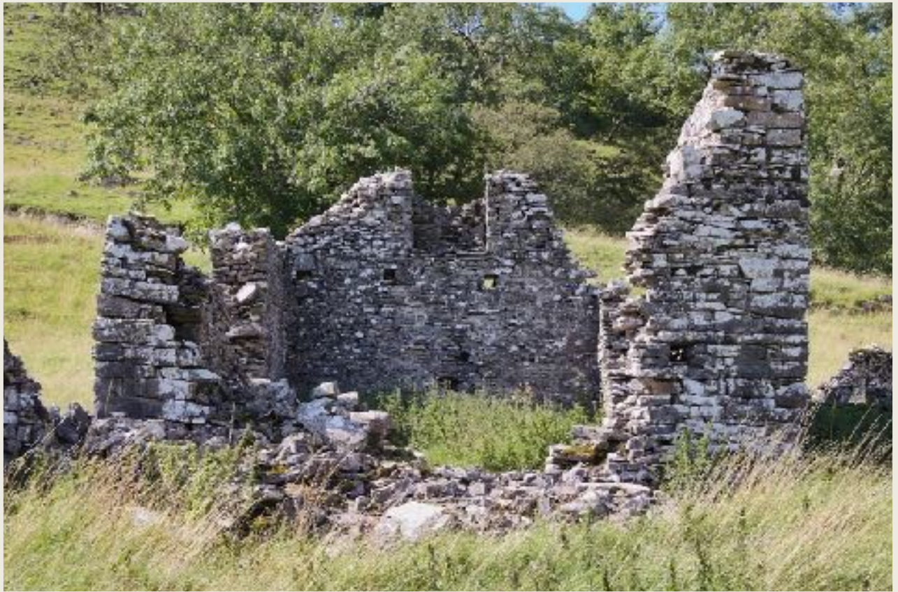
East gable, substantially lost. The unusual construction and steep terrain make it unlikely that there were any openings beyond putlogs and ventilation.
