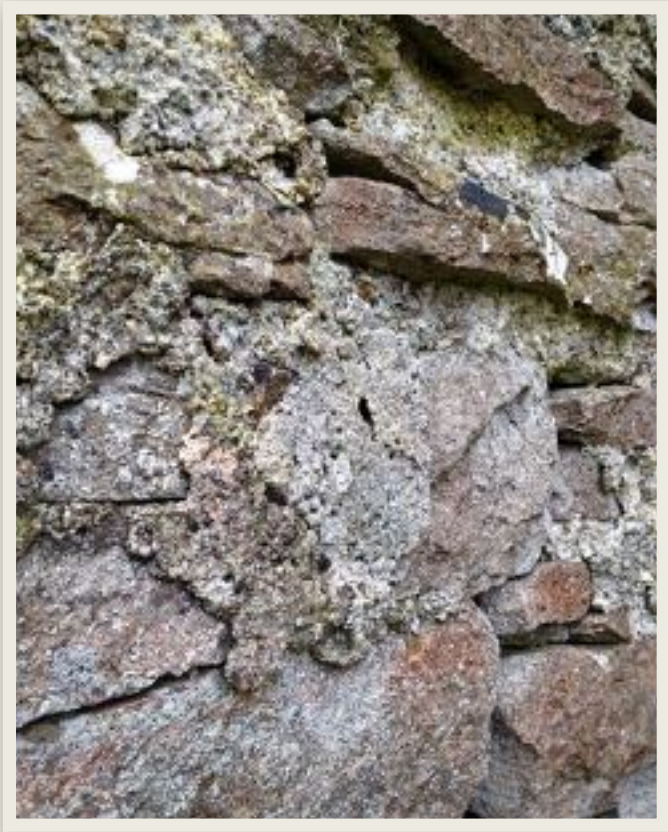
(Top left) Remnants of render-type finish on interior wall, possibly harled (top right & bottom left) remnants of limewash, evidently applied to mortars that were already recessed or eroded.
